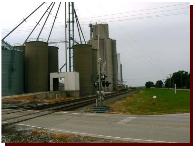
Rail crossing at Milmine
